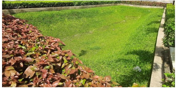
Fig. 4.A photographic view of constructed wetland to store storm water runoff.
