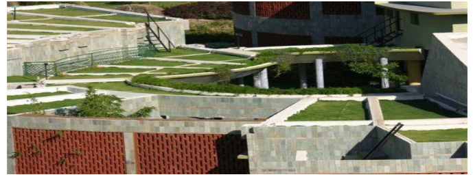
Fig. 1. Photographic view of green roofs at the CII-Sohrabji Godrej Green Business Centre (CIIGBC), Hyderabad, India .
